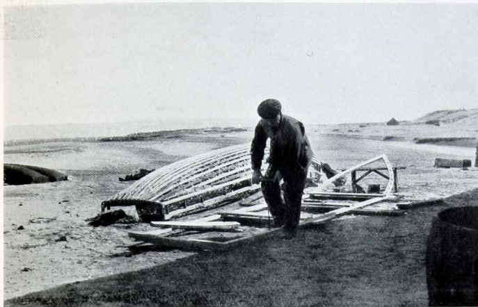
FIG. 1. AN ARAN ISLANDS CURRAGH UNDER CONSTRUCTION Boring holes in the lower gunwale.
