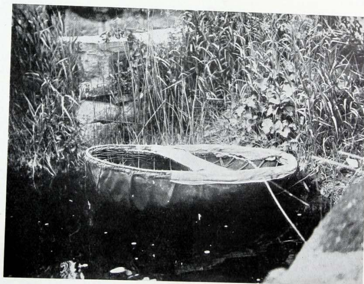
FIG. 2. A BOYNE CURRAGH AFLOAT SHOWING THE CLOTH PROTECTION ON AFTER GUNWALE
